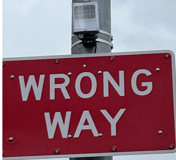
Flood light and LED flashing sign
