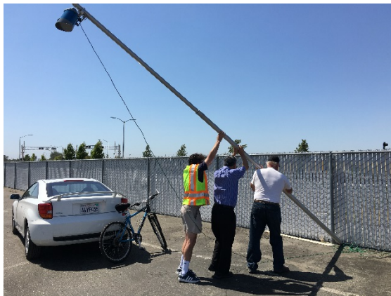
Pole was lowered and mounting height of radar detector raised to 20 feet
