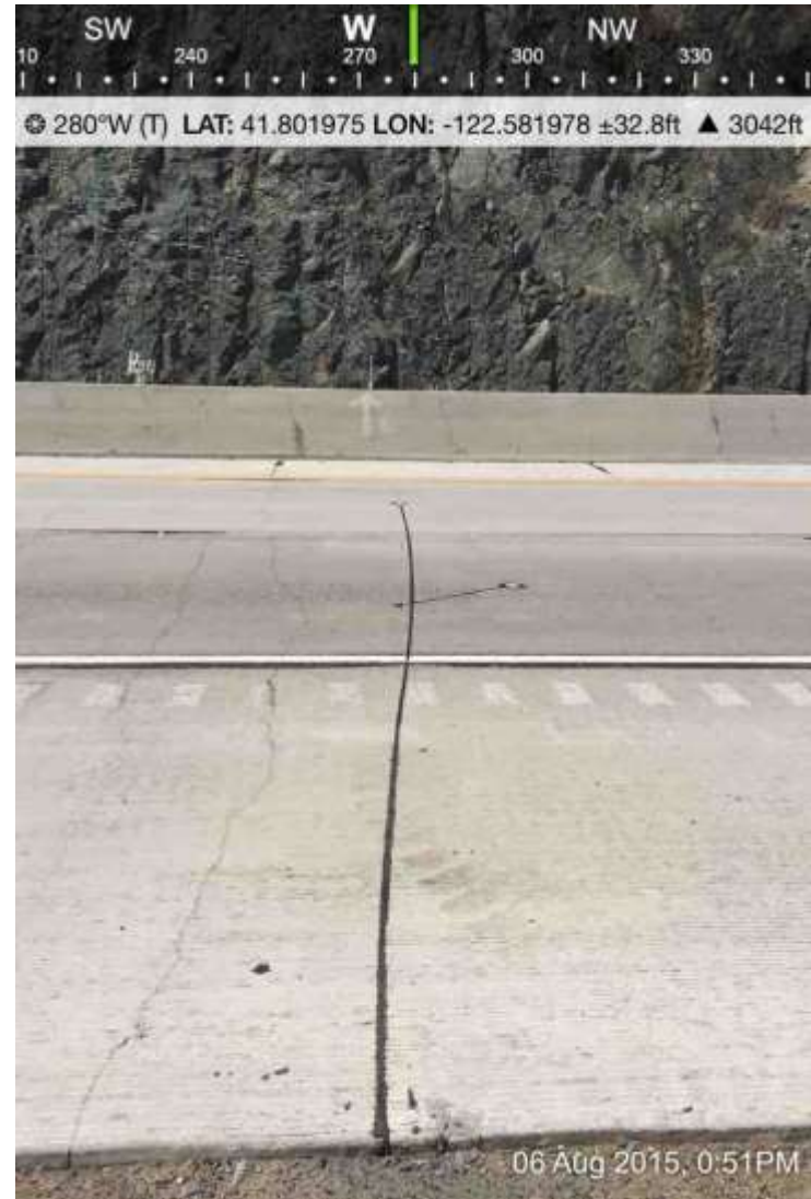
Notice saw cuts for wired power and data.
