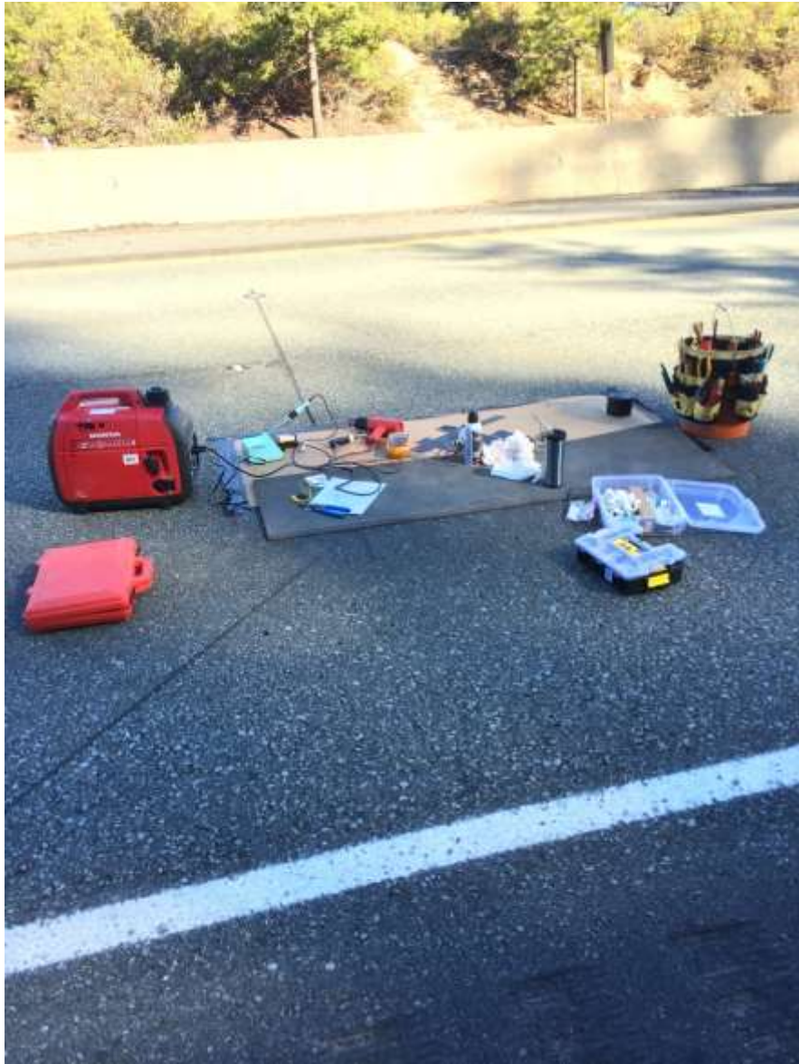
Setting up for work on In-Pavement Sensor. Lane closure on I-5.
