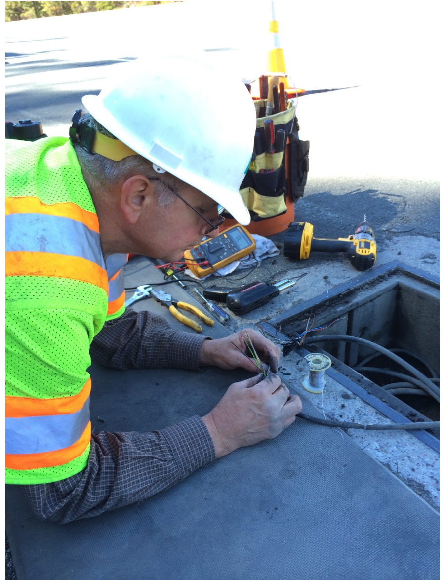
Mike Re-Splicing cable per new Caltrans D2 spec.
